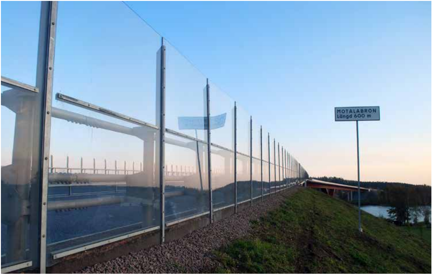
Soundwalls of transparent PC on the Motala bridge.
