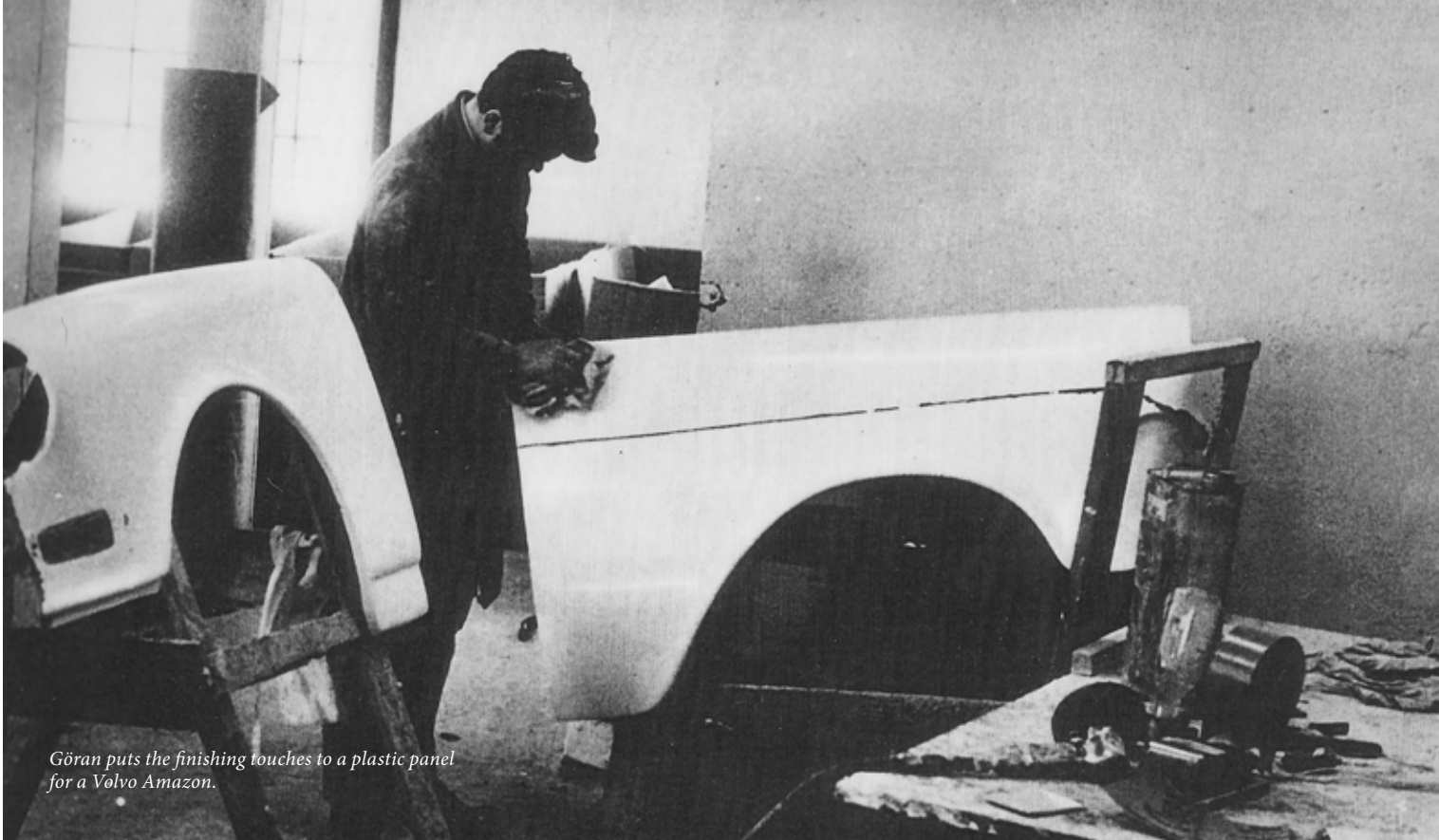
Assembling a plastic panel on a Volvo Amazon.
