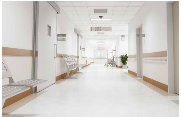
In corridors with a lot of traffic, the walls and corners quickly get worn down.
